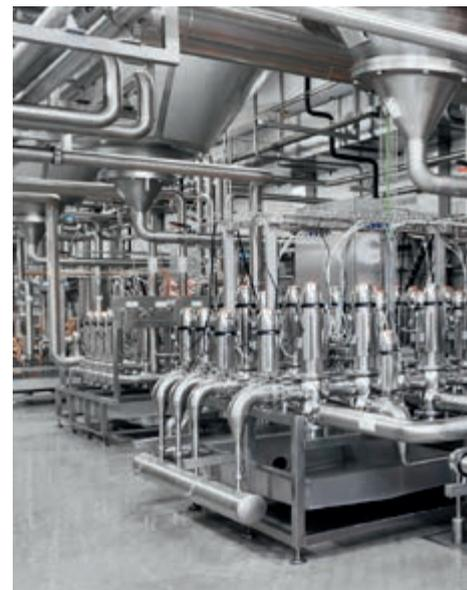
Two-level, fully-automatic valve manifolds with DN125/100 mixproof double seat valves, to connect ten tanks to seven filling lines.
