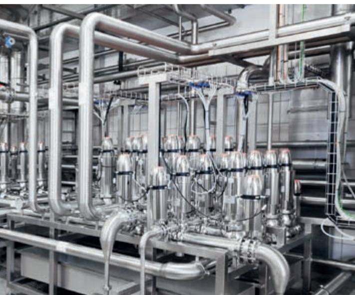
Switch from manual to automated control: In the filter cellar, the panel equipment was replaced by double seat valve manifolds.
